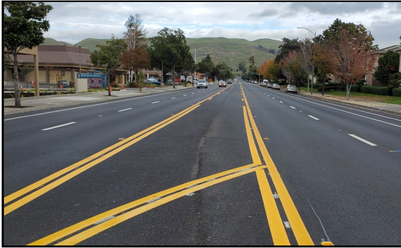
Good (PCI 100 to 70) – Landess Ave PCI 94
