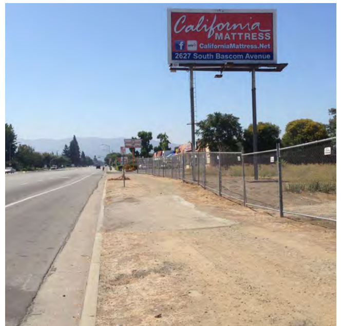
Incomplete sidewalks impede access for pedestrians traveling along the corridor
