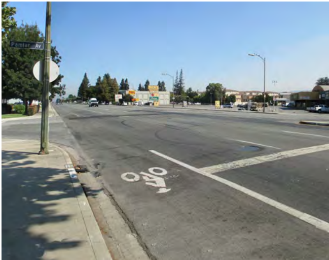
Existing northeast view of South Bascom Avenue at Pamilar Avenue
