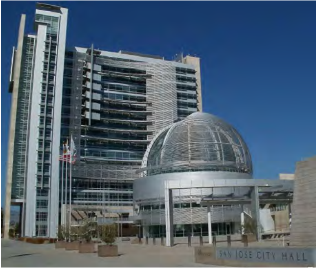
City of San José City Hall
