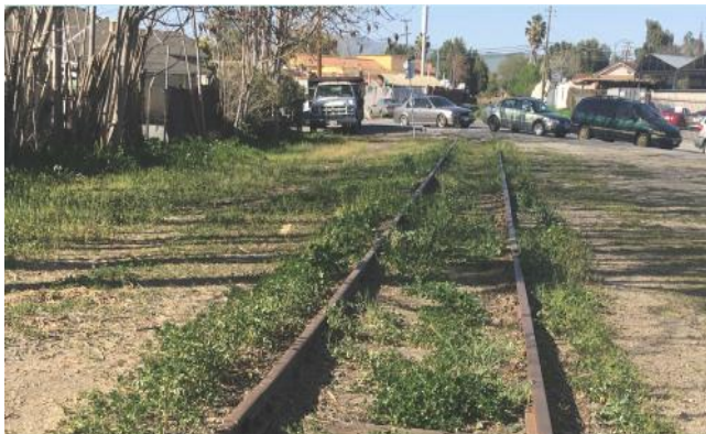
Figure 20: Valley Transportation Authority-owned Tracks that be converted to trail
