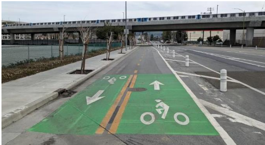
Figure 10: Plastic bollards along the Class IV bikeway on Mabury Road near the Berryessa BART Station will be upgraded using funding from the Quick Strike grant program.
