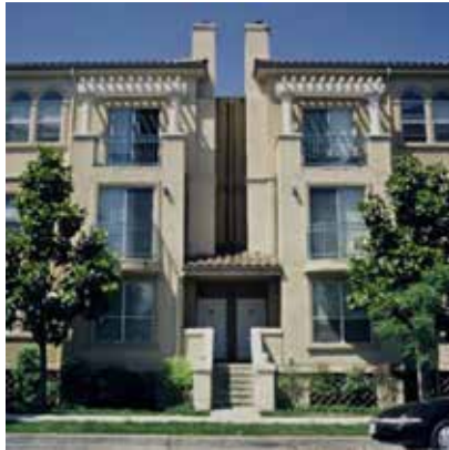
Infill residential building with balconies and trellises
