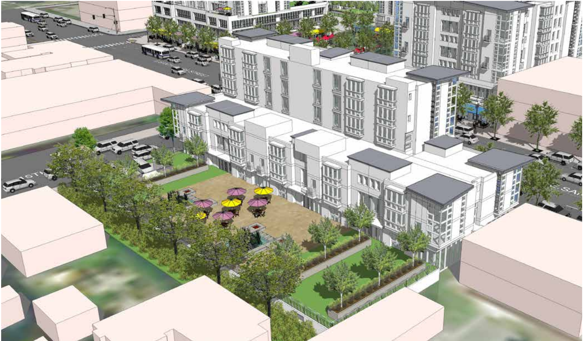
3b: View northwest of mixed-use infill building along East Santa Clara Street, featuring first floor retail space, underground parking, and stepdown next to existing development
