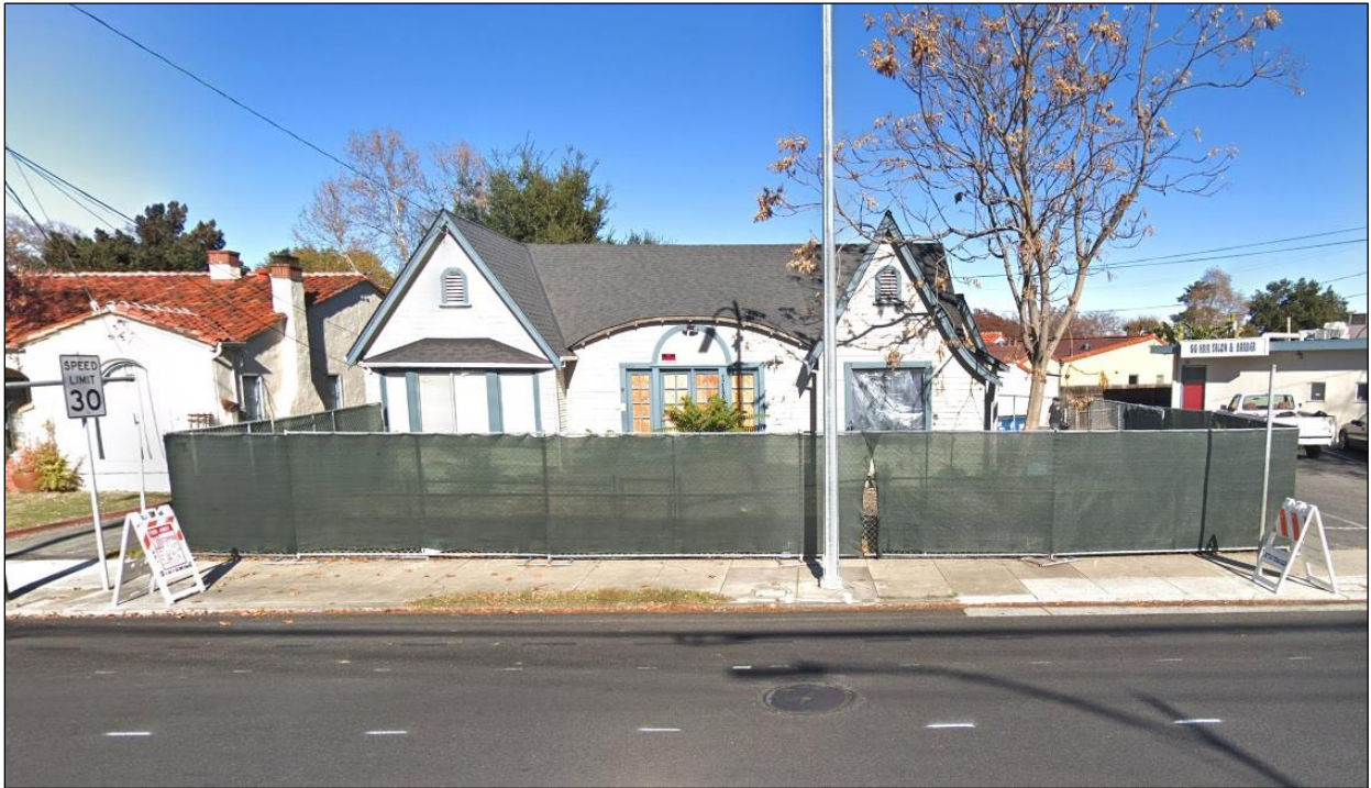
Figure 2: 1131 Park Avenue facing Park Avenue
