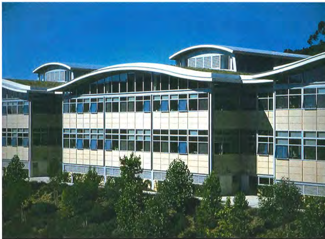
The Gap Inc. headquarters
