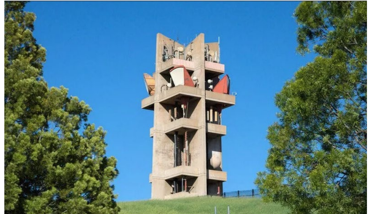
AT&T Tower, constructed 1972
