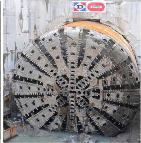
S. Montgomery (eastern) headwall
