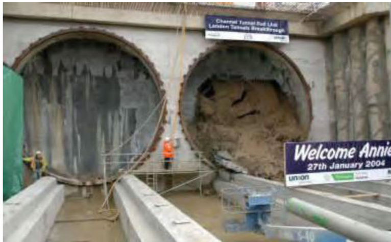
White Street (western) headwall
