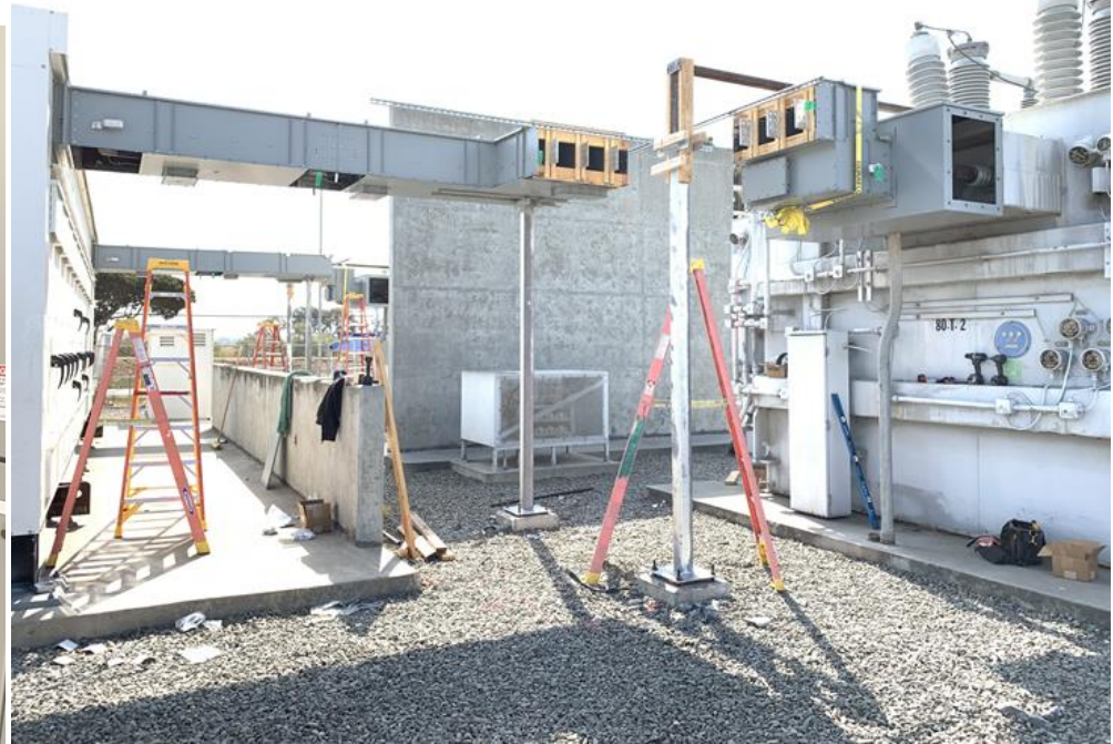
■ Duct installation and supports
