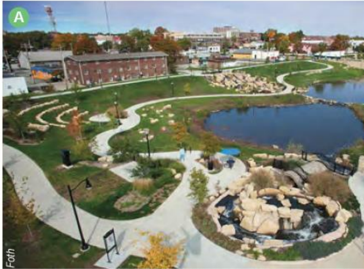
Example of Regional Stormwater Treatment Integrated into Park Setting at Helms Park in Champaign, Illinois
