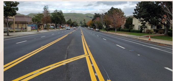
Landess Ave, post-resurfacing 2021
