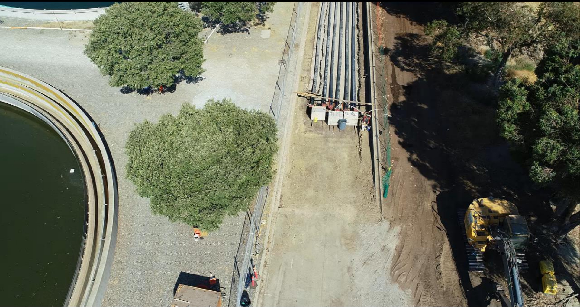
Newly-laid underground pipes
