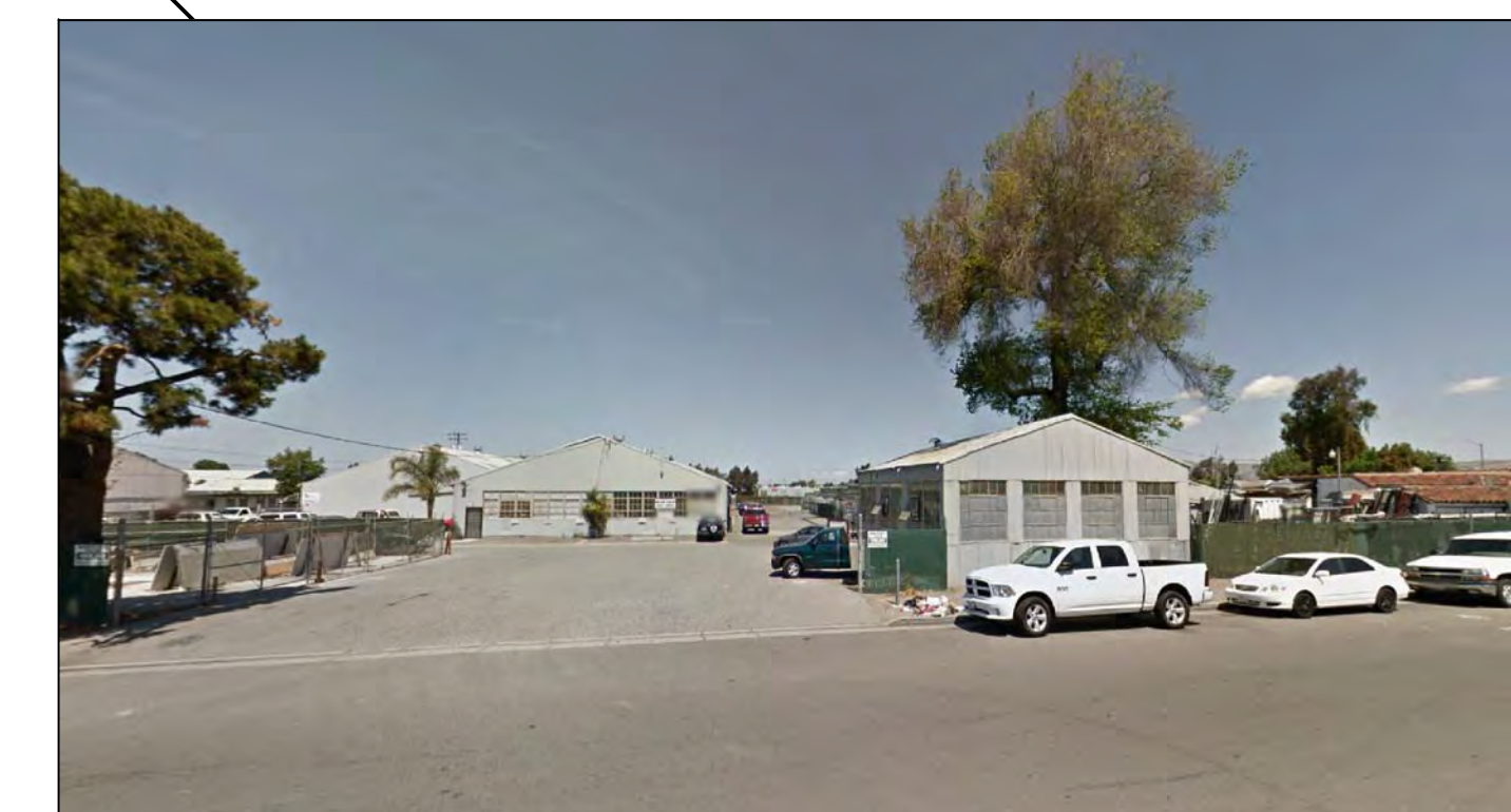
SITE VIEW FROM HORNIN ST.
