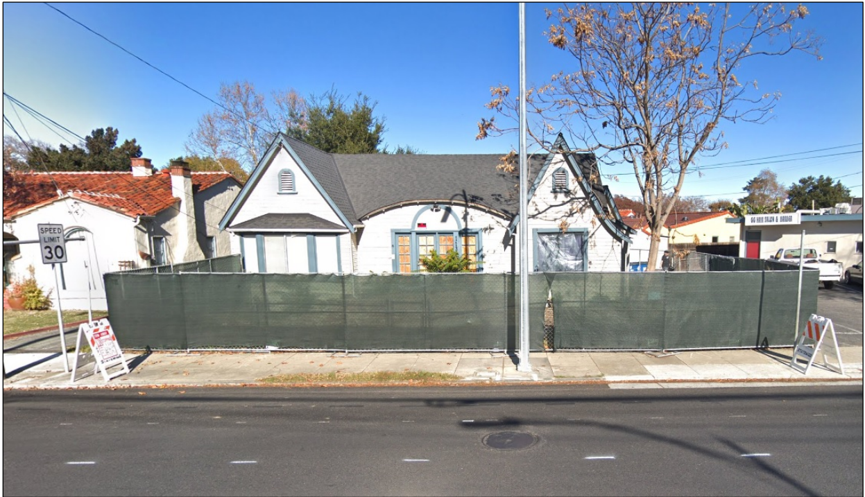
Figure 2: 1131 Park Avenue facing Park Avenue
