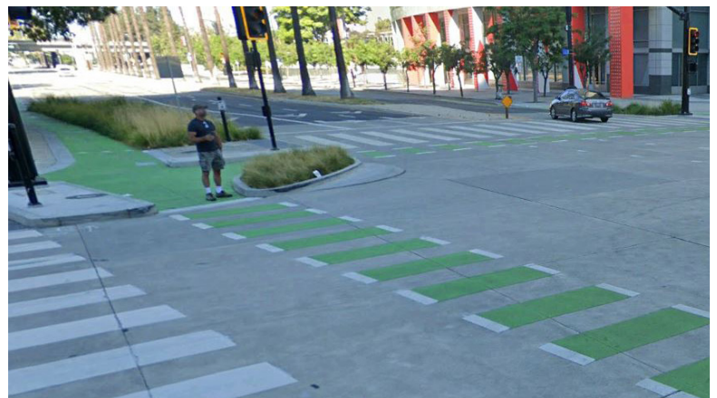
Permanent Protected Intersection at Park Avenue and Almaden Boulevard
