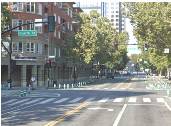
Quick Build Protected Intersection at S 4th Street and San Fernando Street
