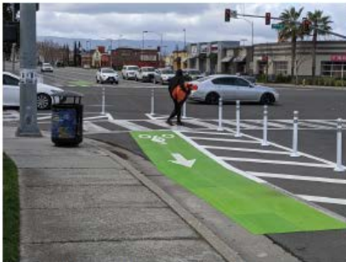
Protected Bike Lane: Painted buffer with bollards provides visible separation and more comfort for cyclists.
