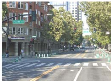
Quick Build Protected Intersection at S 4th Street and San Fernando Street
