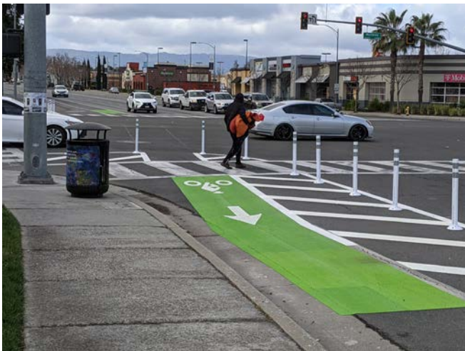
Protected Bike Lane: Painted buffer with bollards provides visible separation and more comfort for cyclists.
