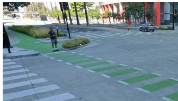
Permanent Protected Intersection at Park Avenue and Almaden Boulevard
