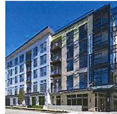
Ground floor design should reflect the building's structural framework, with surface materials, windows, and other elements designed to vary with the structural bay spacing.
