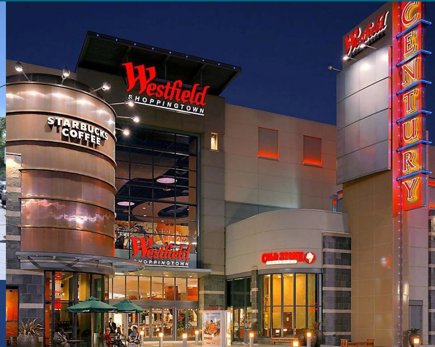
Photo: Fruitdale Station (left), Oakridge Mall
