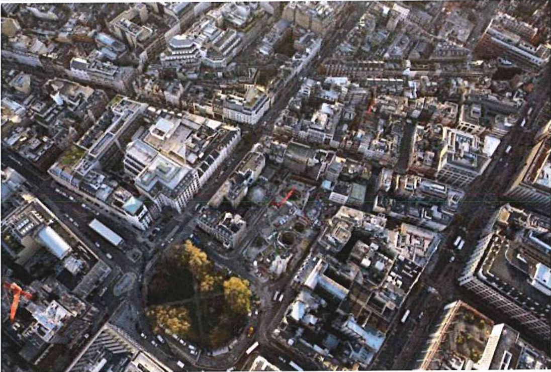
Eastern ticket hall under construction
