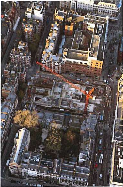
Western ticket Hall under construction
