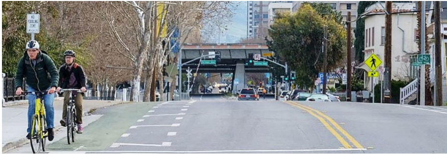
Bicyclists using a buffered bike lane along West San Fernando Street. Source: www.Bikesanjose.com
