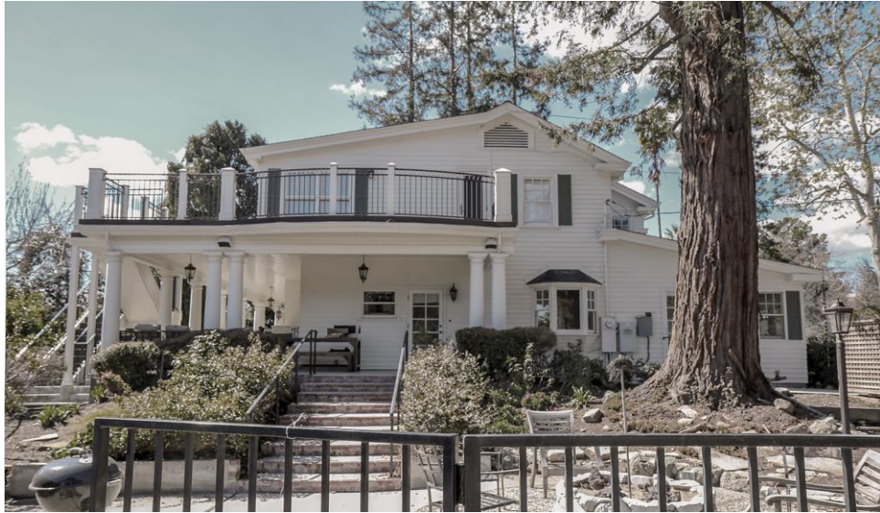
Eastern side of the house. The side door and the sashed window beside it and the attic vent are original. The pillared wraparound terrace and extended back of the house were added during renovations that occurred between 2008-1010.
