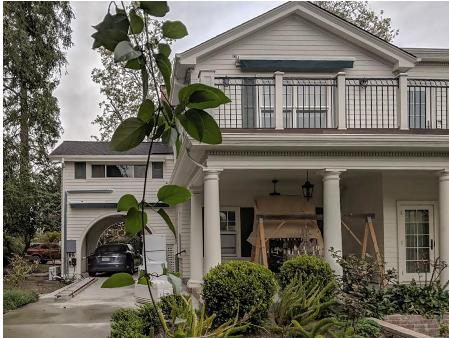
Back of house with port-cochère. View facing north.
