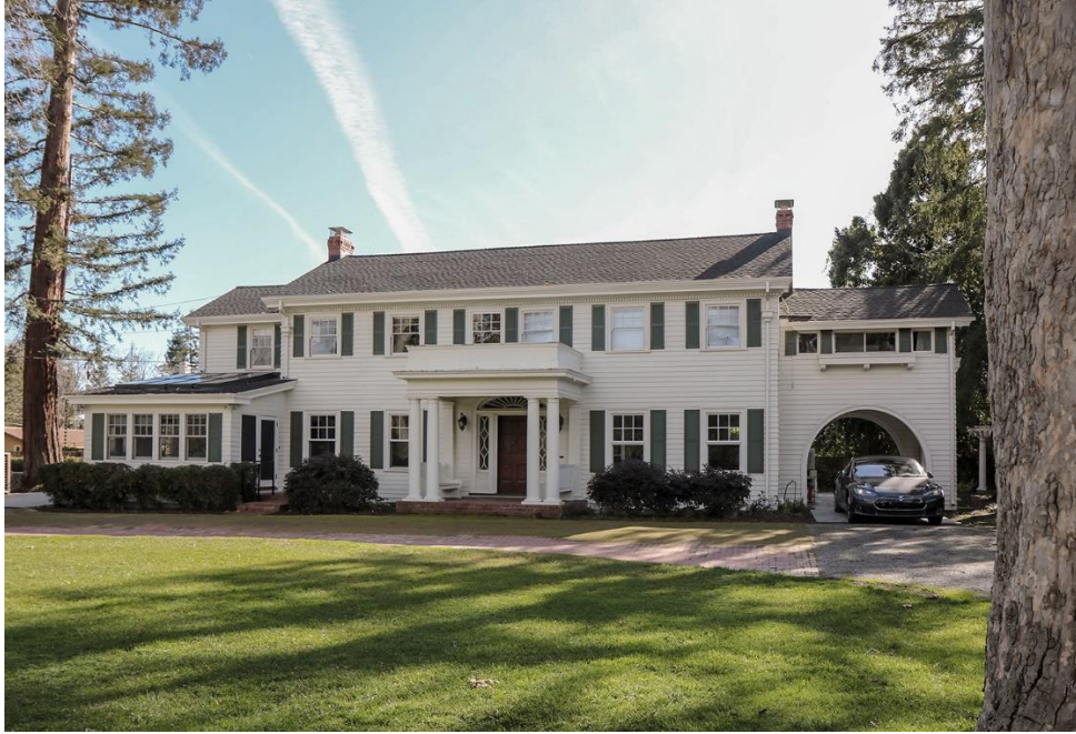
Front elevation viewed facing south-southeast. The distinctive porte-cochère with arched entrances is original to the house.
