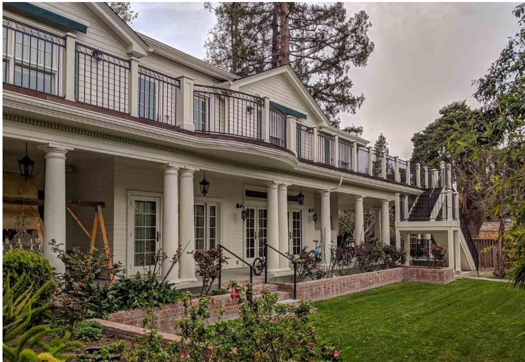
Back of house, view facing northeast, extension of house and added wraparound terrace and staircase.
