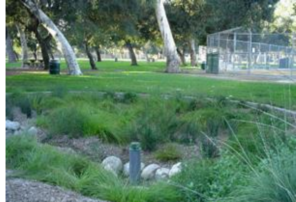
Figure 4. Sun Valley Park vegetated swales in Los Angeles County, California. (Source: U.S. EPA)
