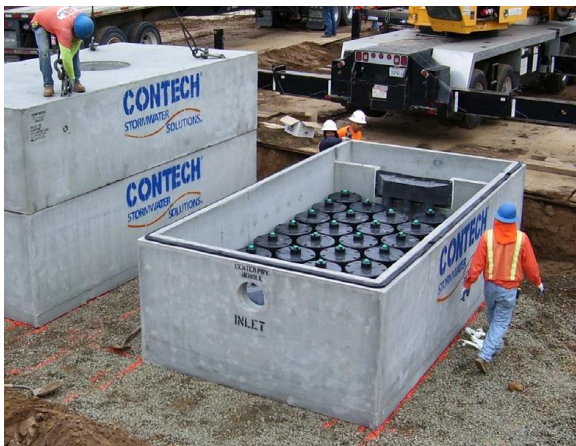
Figure 5. Alta Vista Park underground storage system in City of Redondo Beach, California. (Source: Contech Engineered Solutions)
