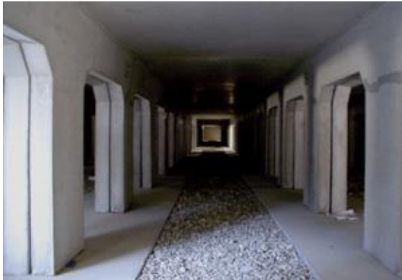
Figure 3. Sun Valley Park underground infiltration gallery in Los Angeles County, California. (Source: U.S. EPA)
