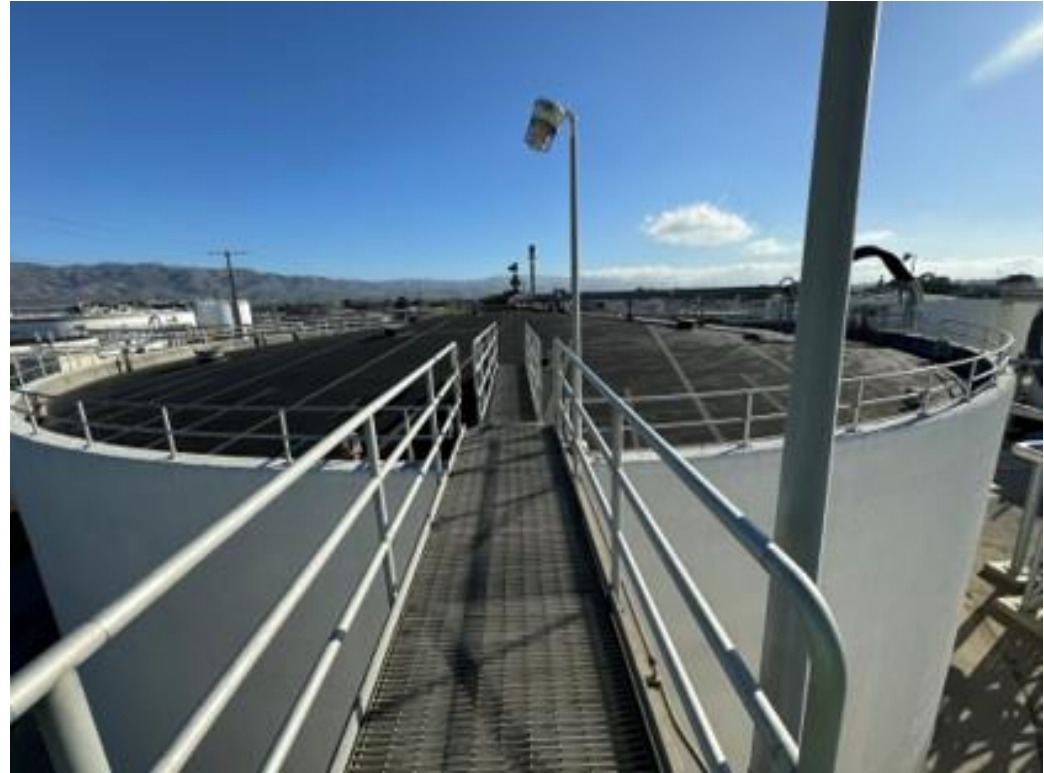
One of the four mesophilic digesters slated for upgrade as part of the Additional Digester Facility Upgrade project
