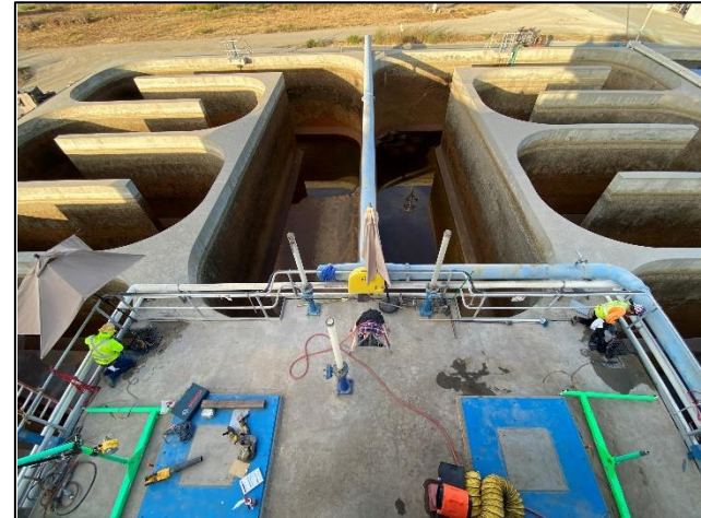
Serpentine chlorine tank rehabilitation work
