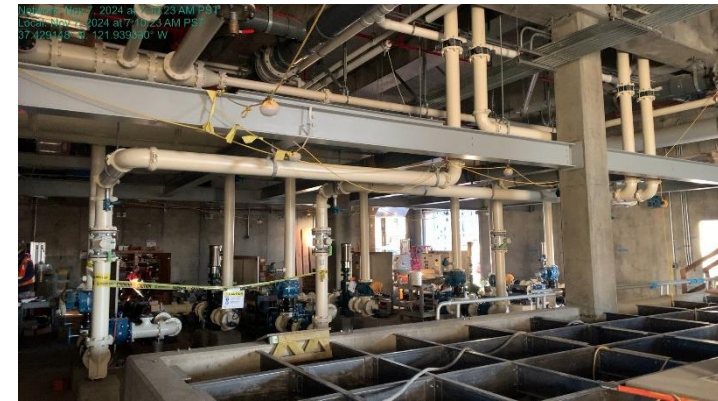
Centrifuge feed pumps and piping installation
