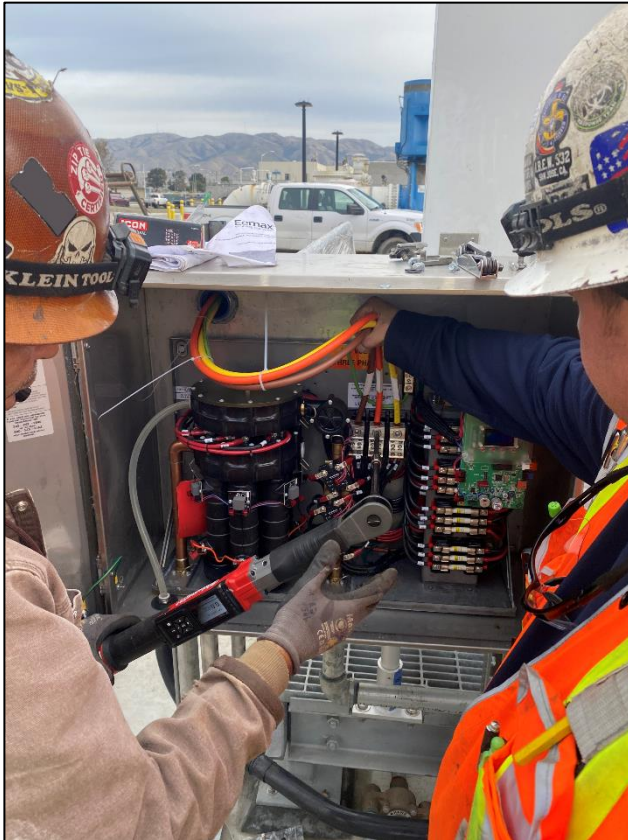
Staff performing torque test for power feed into new eyewash station
