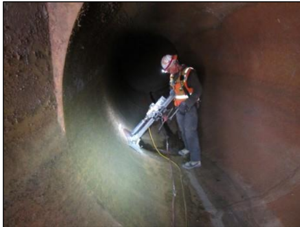
Pipe condition assessment for the Yard Piping Improvements - Phase 3 project
