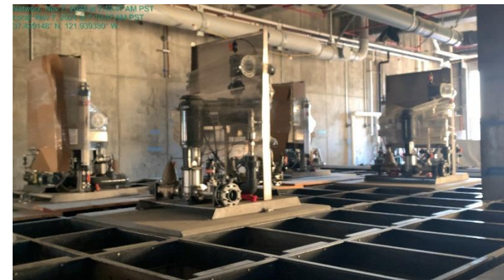
Blend units activate polymer to support dewatering
