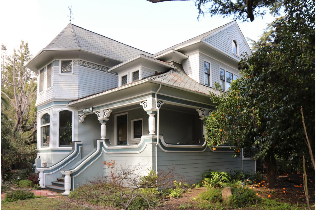
Southern and eastern elevation viewed with camera facing north.
