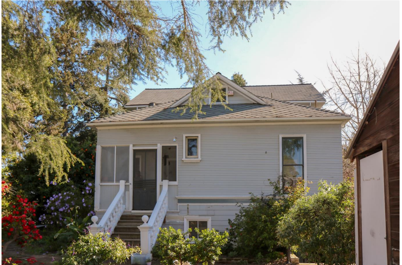
Northern (back) elevation viewed with camera facing south-southwest. The porch was enclosed at an earlier unknown date. The current owners added the railing on the back steps.
