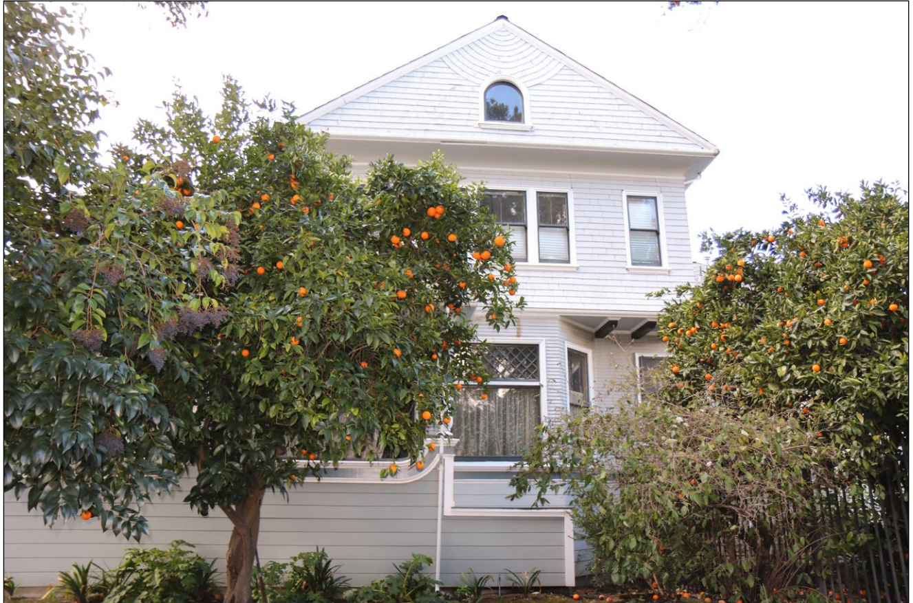
Eastern elevation viewed with camera facing west-northwest.
