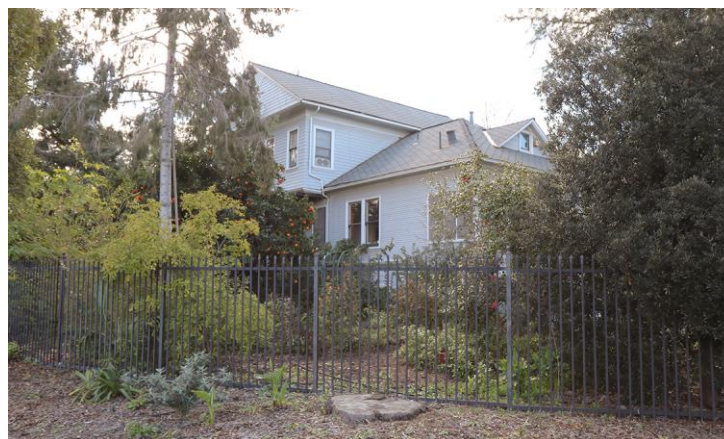
Eastern elevation and back wing viewed with camera facing southwest.
