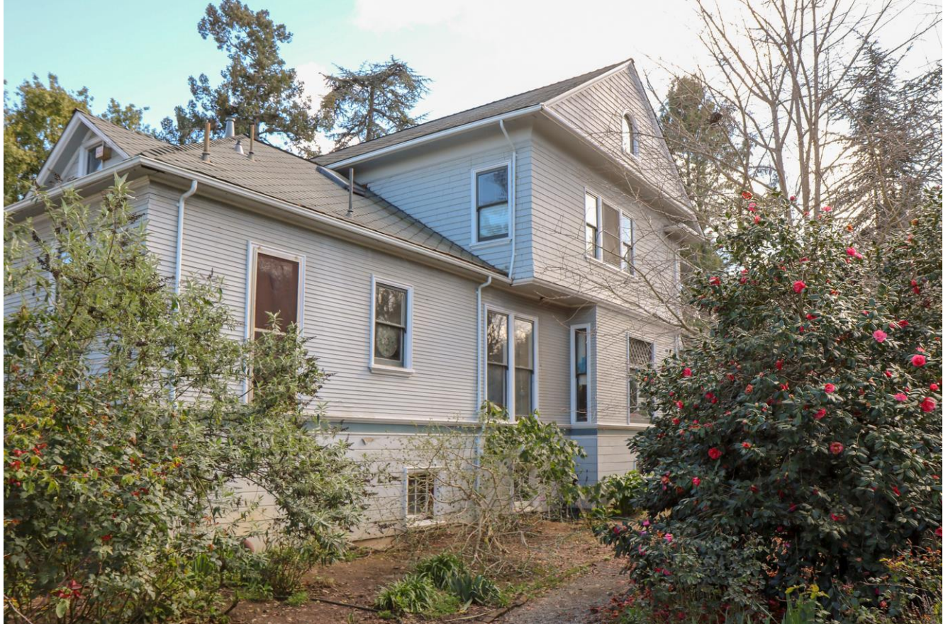
Western elevation viewed with camera facing south.
