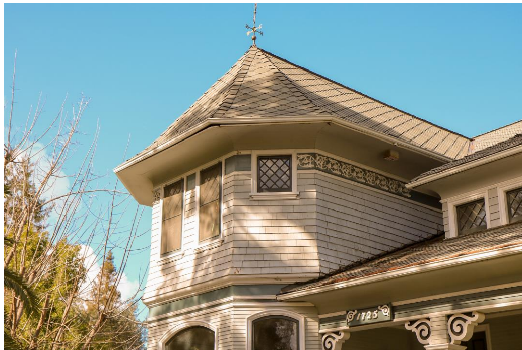
Tower roof closeup.
