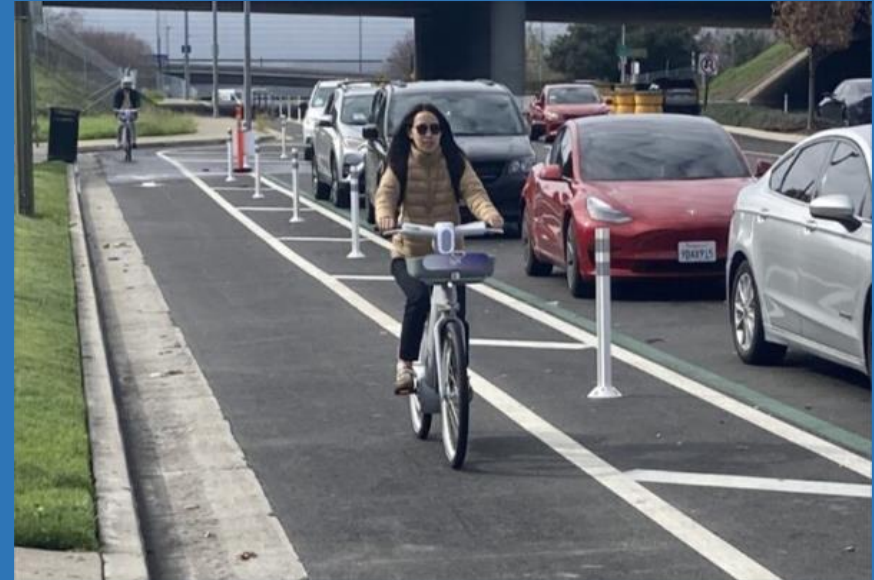
Parking-Protected Bikeway on Airport Pkwy
