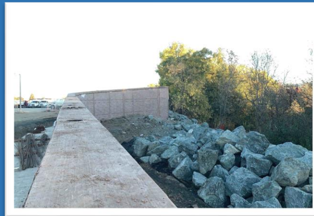
Retaining Wall for Project 1
