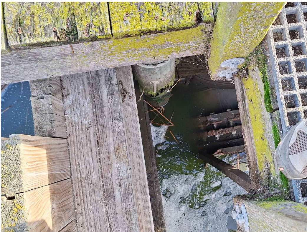
Photo: North Pile (no. 1) is cracked
