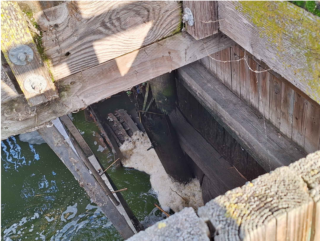
Photo: Center Pile (no. 2) is split
