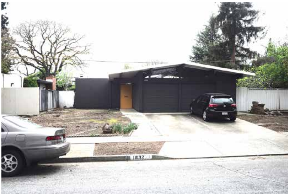
Fairglen Additions Santa Clara County, CA Photo 13 of 20 (SJ-1184) (115)
