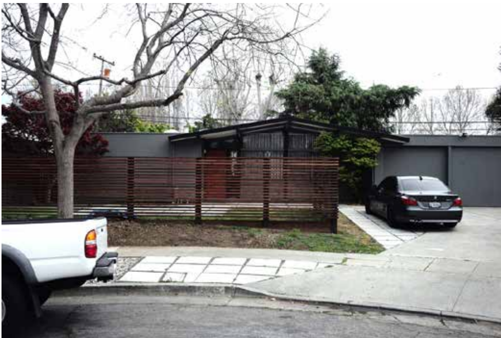
Fairglen Additions Santa Clara County, CA Photo 12 of 20 (SJ-1163) (187)
