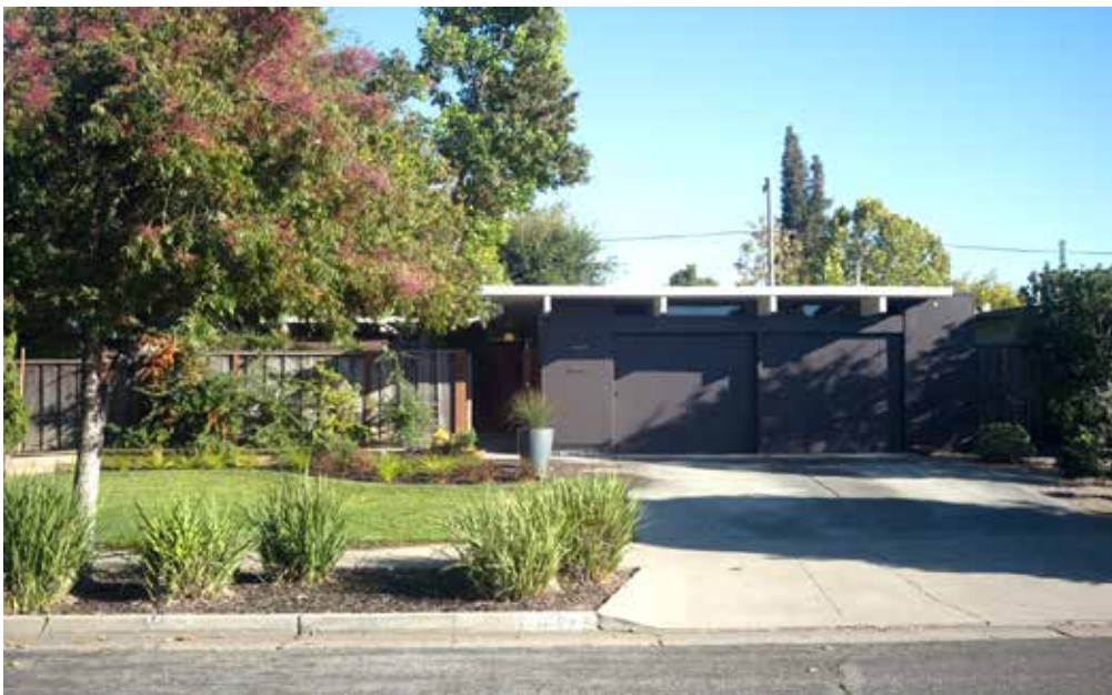
Fairglen Additions Santa Clara County, CA Photo 16 of 20 (SJ-24) (118)
