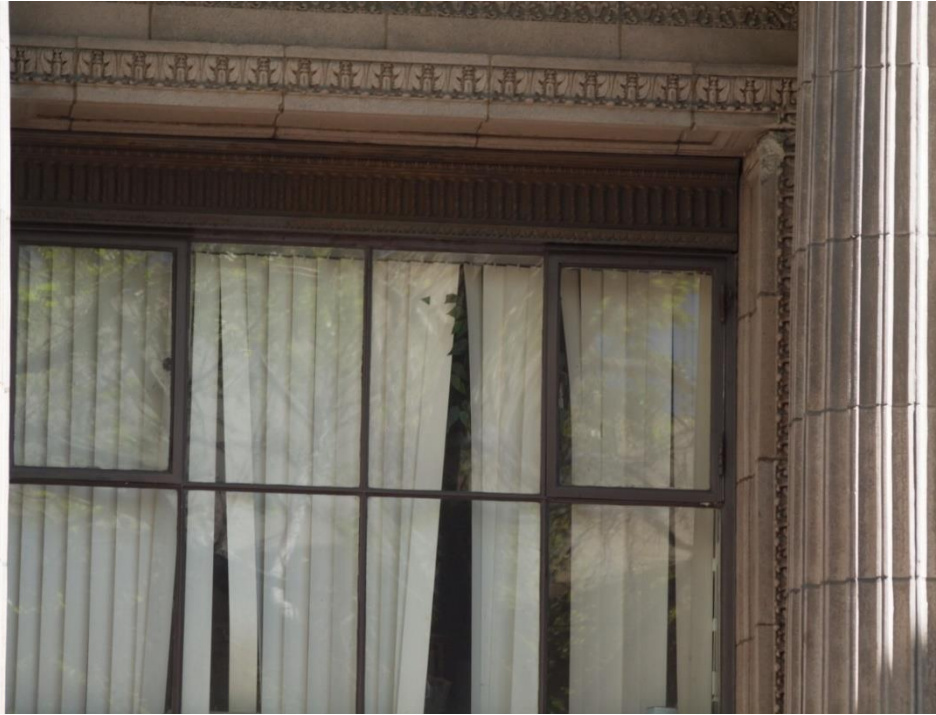
Detail view of storefront windows at base to remain
