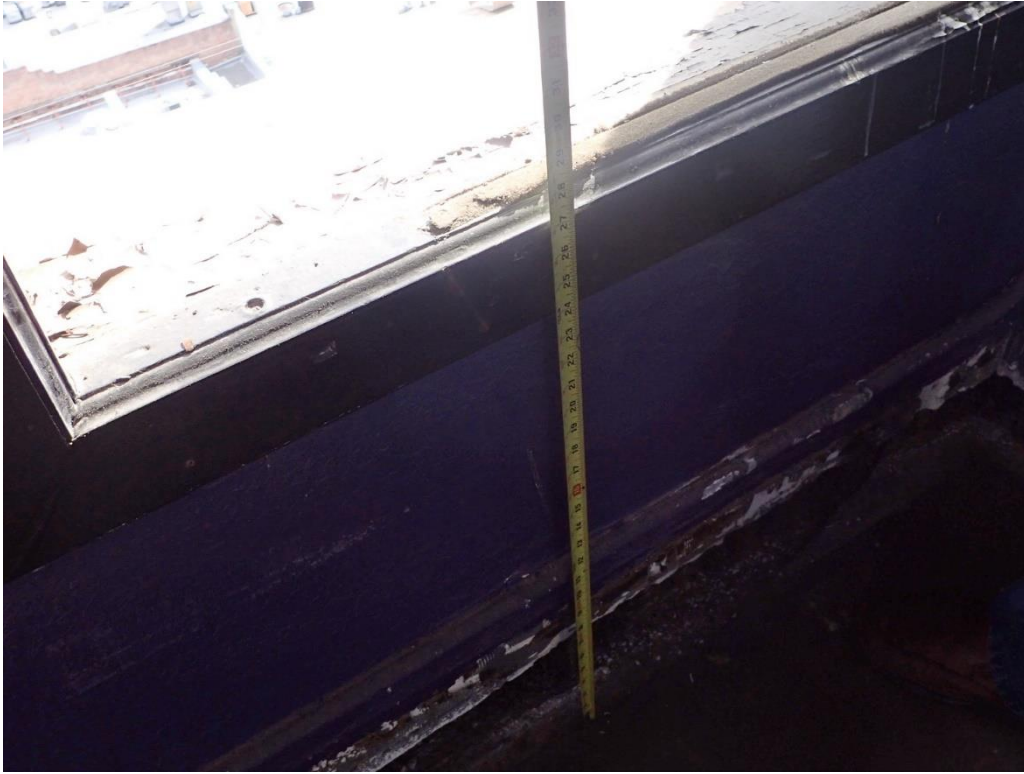
Interior sill height
