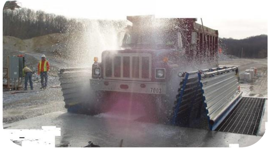
Installed wheel wash systems to ensure runoff into waterways are clean
