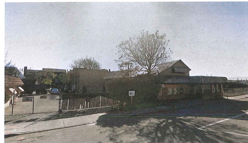
Project Location View B
