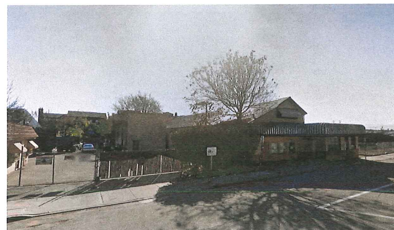
Project Location View B
