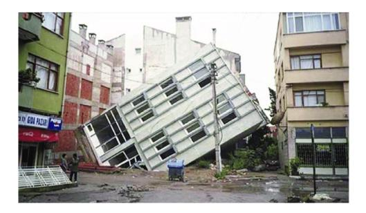
And here (picture below) is a taller building damaged in Taiwan by a 2018 liquefaction event:
