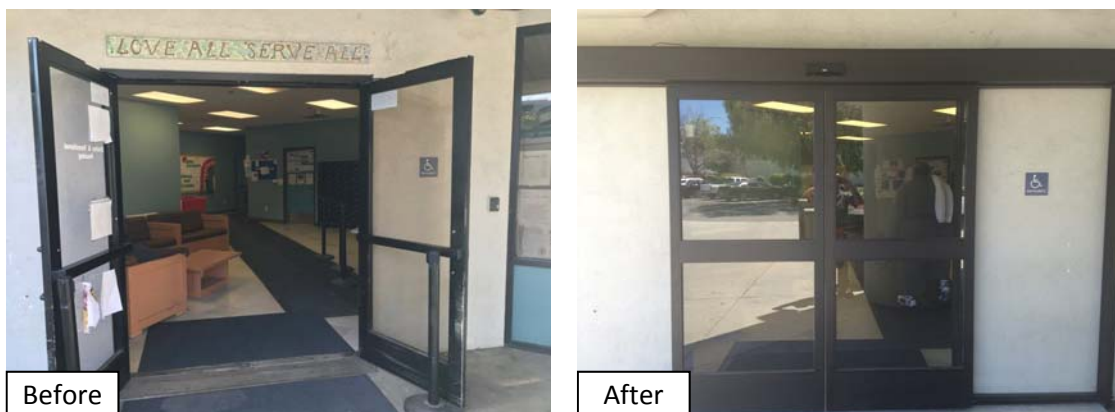
ADA Accessibility Improvements at BRC Homeless Shelter
