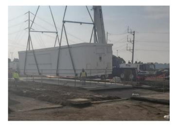
Switchgear being laid onto pad
