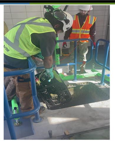
Contractor deploying remote operated vehicle to perform condition assessment in the 108-inch Filter Influent pipe in the Yard Piping Improvements – Phase 3 project
