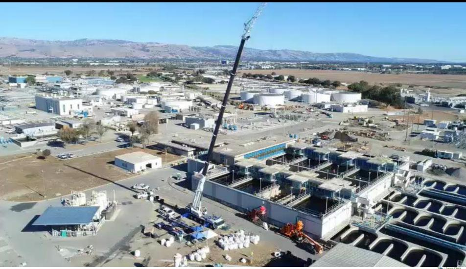
New gravel in the white sacks being added to the Filter Building as new media
