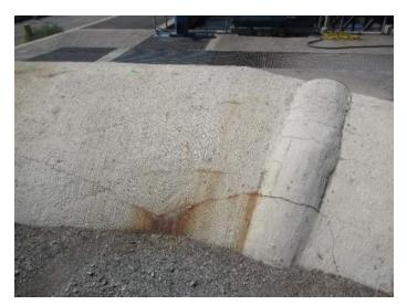
Corrosion and cracking of the 96" raw sewage pipe that will be rehabilitated by the Yard Piping Improvements – Phase 2 project
