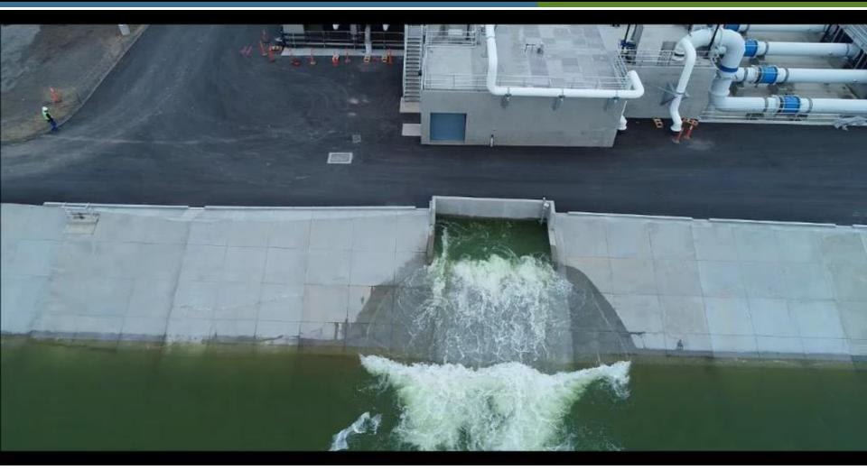
Flow circulates in a loop through new Headworks, Emergency Overflow Basin and EBOS
