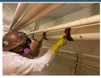
Demolition of Surface Wash line containing lead paint in Gallery A
