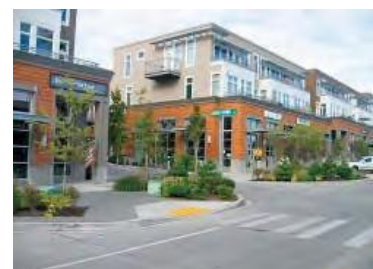
Enhanced Crosswalk with Bulb out Source: Bike Ped Images, 2010
