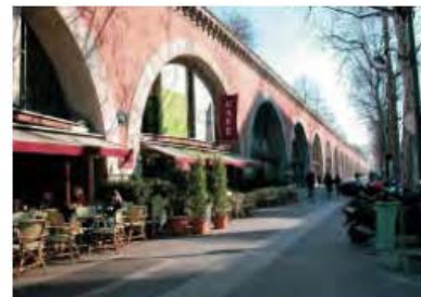
The elevated railway structure can include ground floor uses that activate the street level.
