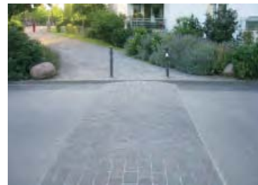
Speed tables work to both slow down traffic as well as provide a clear pathway way for pedestrian travel. They can be adopted for both residential and urban conditions.
