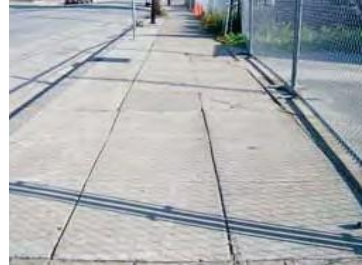
Existing Conditions, Montgomery Street Source: Fehr & Peers, 2010
