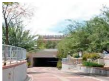
Enhanced Underpass, Arizona Source: Bike Ped Images, 2010
