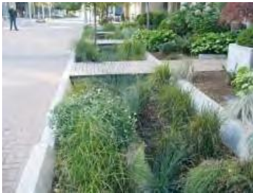
Bioswales retain rain water and reduce the impact on the storm water system. If designed well, they can improve and green the streetscape.
