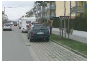
Permeable paving for street parking strips reduces rain water run-off.
