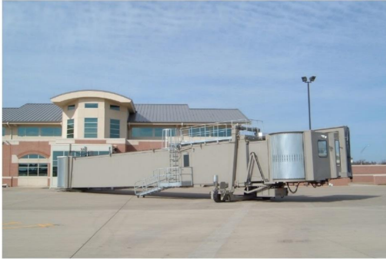
Photo 1: Example of a Radial Boarding Bridge
