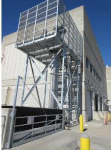
Figure 1: Biosolids receiving pit and conveyance
