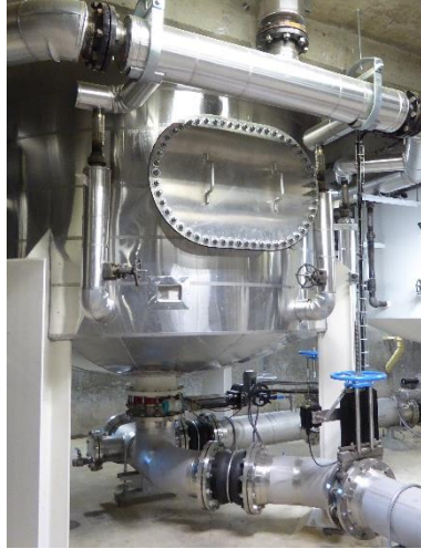
Figure 3: Lystek THP Reactor at the Fairfield OMRC
