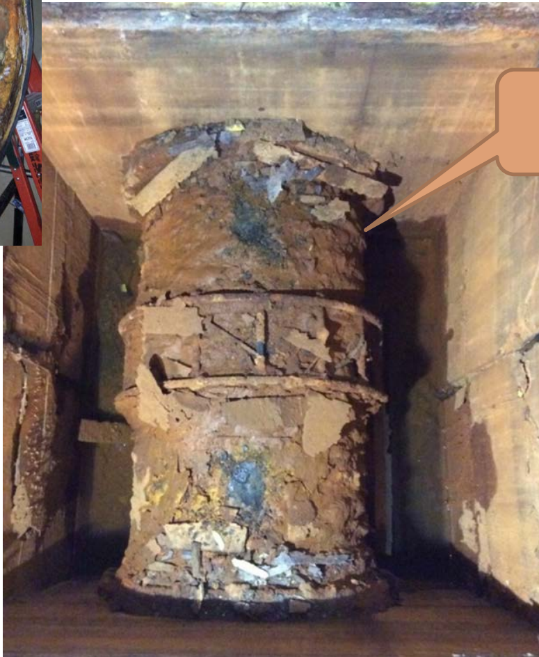
Corroded Piping
