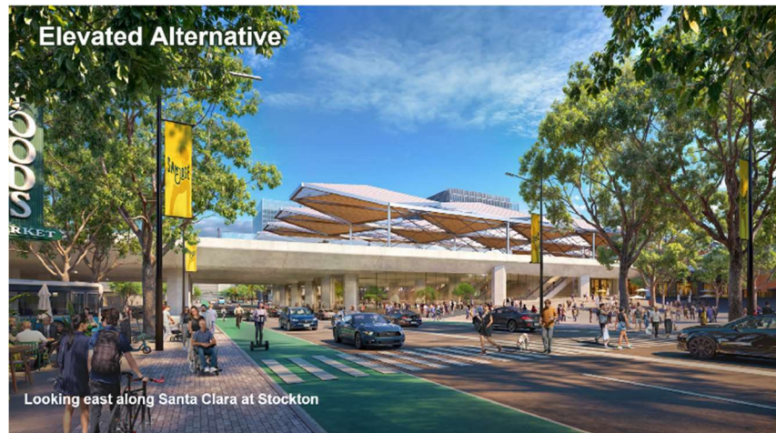
Figure 4 - Elevated Alternative. This option elevates the tracks roughly 25 feet above the surrounding street level to provide better street connections through the station and across the tracks. This option is most like the 2020 Concept Layout.
