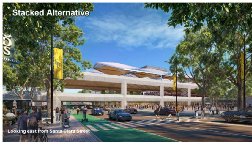
Figure 5 - The Stacked Alternative. This option allows for a narrower station footprint by putting high-speed rail on a higher platform level above the other heavy rail modes. The Partner Agencies discarded this option in August 2024 considering engineering and constructability concerns, as well as its perceived visual impacts on neighborhoods west of the station, as shown in this rendering.
