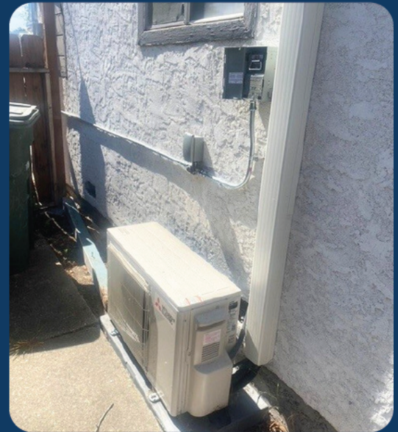
Figure 1: Typical Retrofit Condenser Installation
