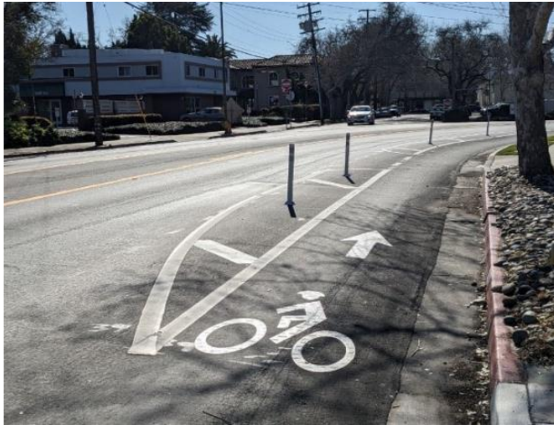
Left: Lane reduction and new bike lanes on Taylor St. implemented via pavement maintenance.
