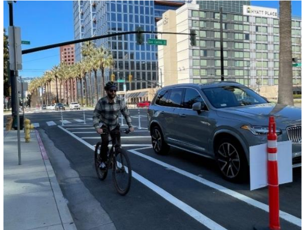
Right: New protected bikeway on Almaden Blvd. upgraded from existing bike lanes during paving.
