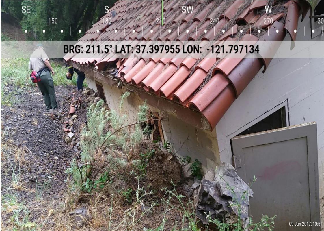
Restroom at Alum Rock Park
