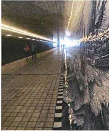
Figure 4: Amsterdam Centraal Station Passageway
