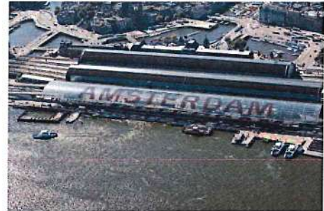
Figure 2: Amsterdam Centraal Station
