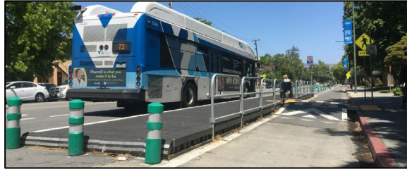
Transit Boarding Island
