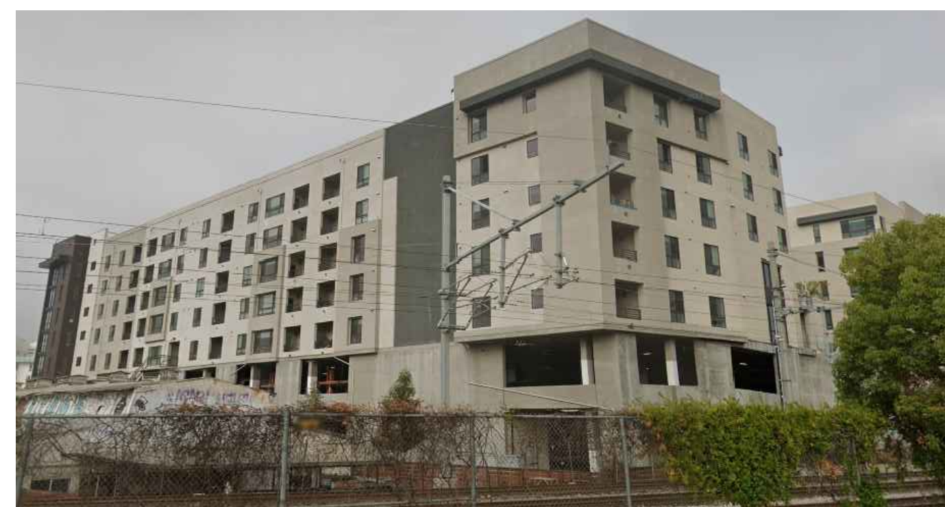
5 NORTH-EAST VIEW FROM MONTGOMERY ST. PARKING LOT
