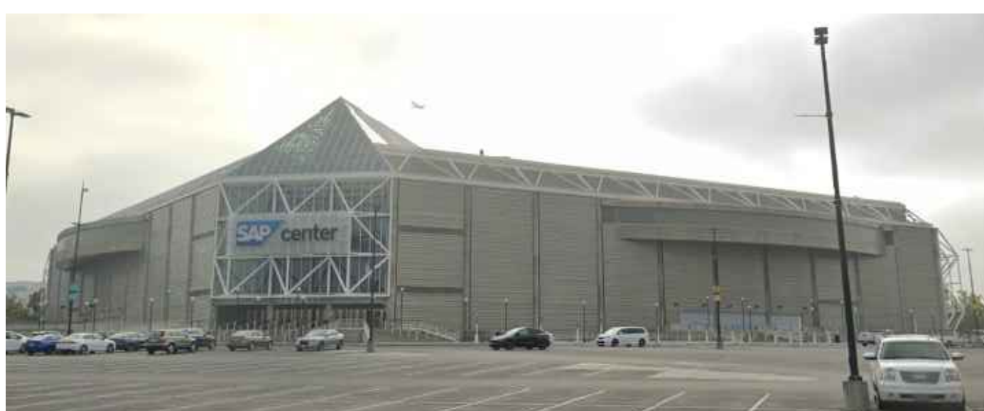
9 NORTH-EAST VIEW FROM MONTGOMERY ST. PARKING LOT
