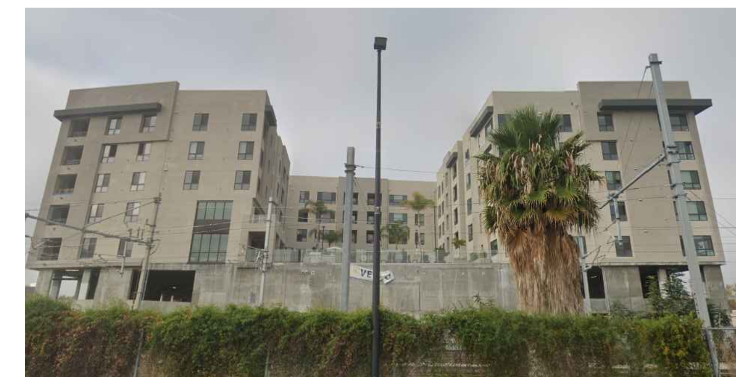
6 NORTH FACADE VIEW FROM MONTGOMERY ST. PARKING LOT
