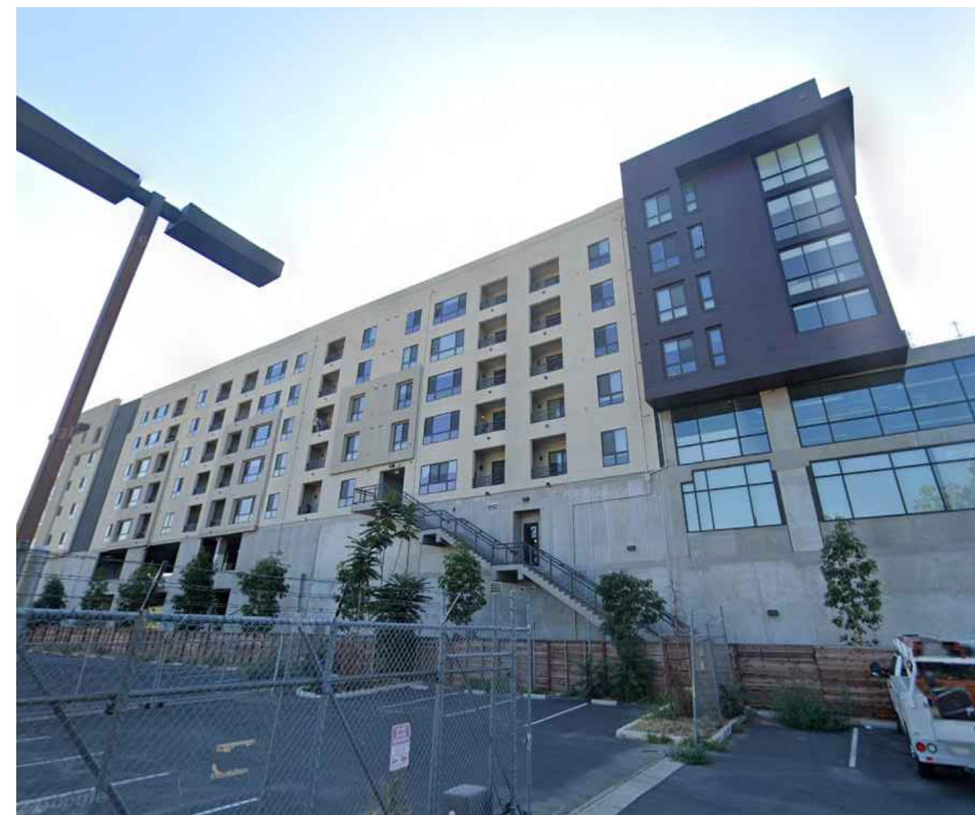
3 WEST VIEW FROM STOCKTON AVE.
