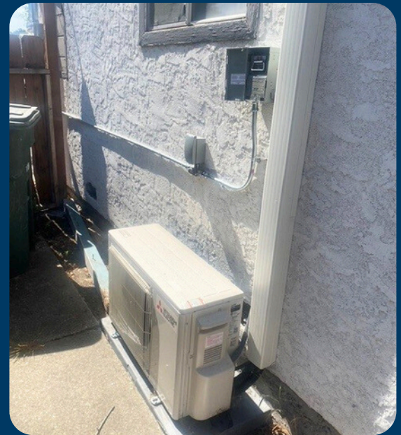
Figure 1: Typical Retrofit Condenser Installation
