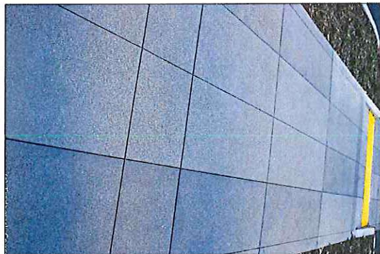
A SAWCUT CONCRETE WITH LIGHT SANDBLAST
