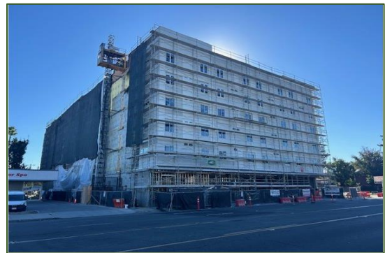
Image 15 Affordable housing 2350 S Bascom Ave (Under Construction)
