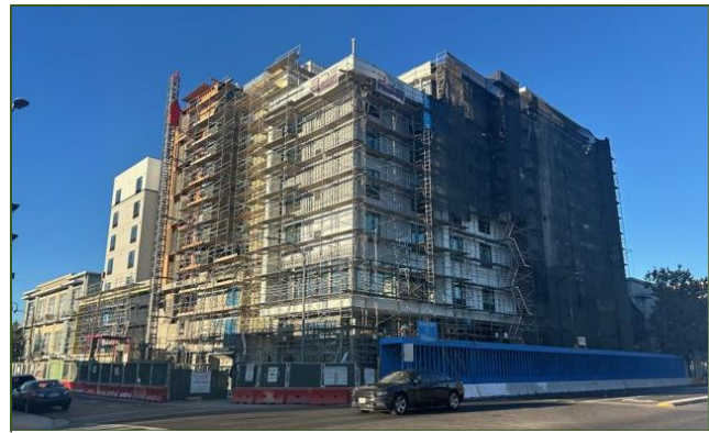
Image 24 Marriot Keystone Hotel at 495 W. San Carlos Ave (under construction)
