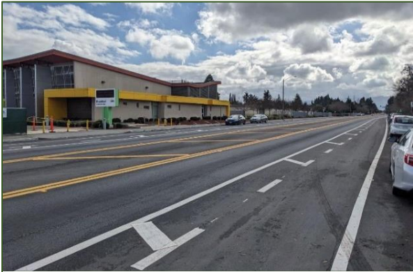
Image 21 New bike lanes on Leigh Ave near Blackford Elementary
