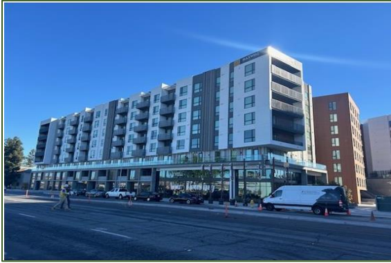
Image 13 Signature project 1350 S Bascom Ave residential building (under construction)
