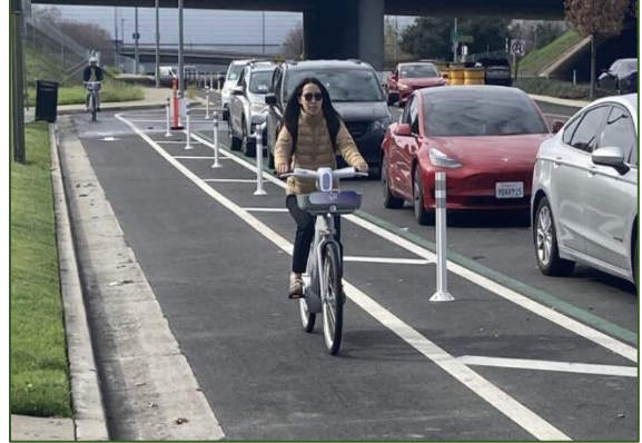
Image 20 Protected bikeway on Airport Parkway implemented through pavement maintenance
