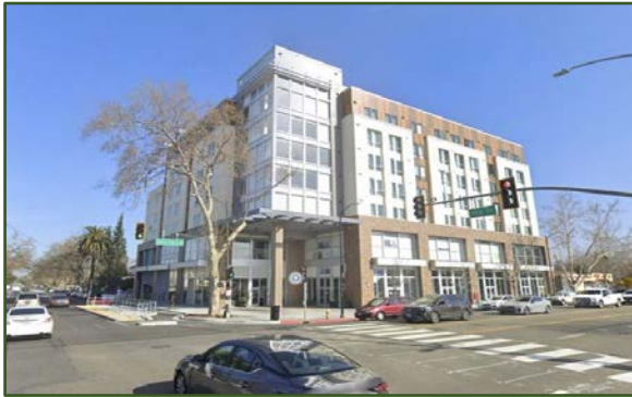
Image 11 Sparta student housing (construction complete in 2022)
