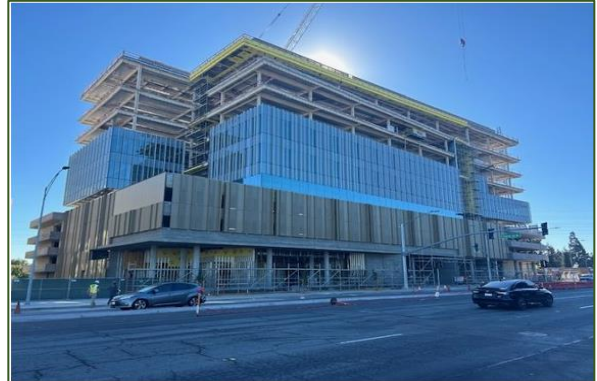
Image 14 Signature project 1350 S Bascom Ave office building (under construction)
