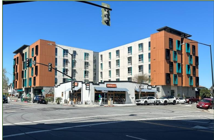
Image 23 Affordable housing project at 427 Auzerais Ave (construction complete)
