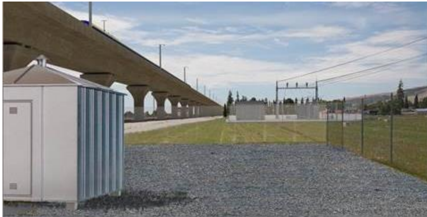
Alternatives 1 and 3 traction power facility on agricultural land
