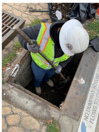
Installing inlet-based full trash capture
