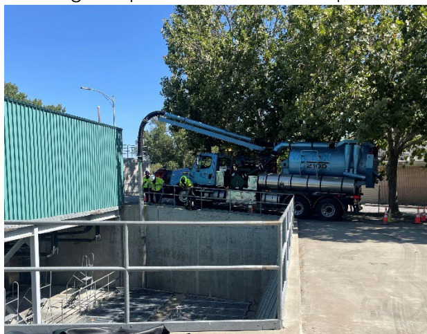
Wet well cleaning of the Oakmead Pump Station
