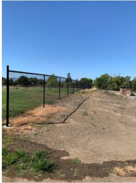
Fencing installations at Tully Minor Ballfield, including 150 feet along the foul ball line and a 70-foot perimeter enclosure, to deter encampments near Coyote Creek.
