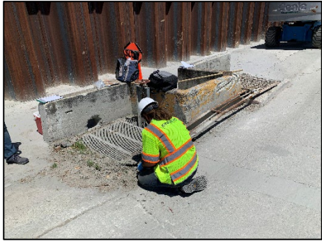
Sampling storm drain catch basins at a potential PCB source property.
