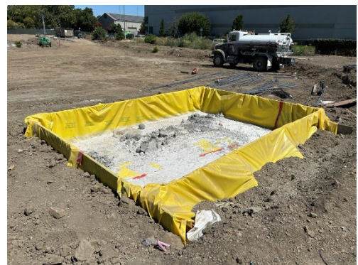
A properly lined and installed concrete washout at an active construction site.
