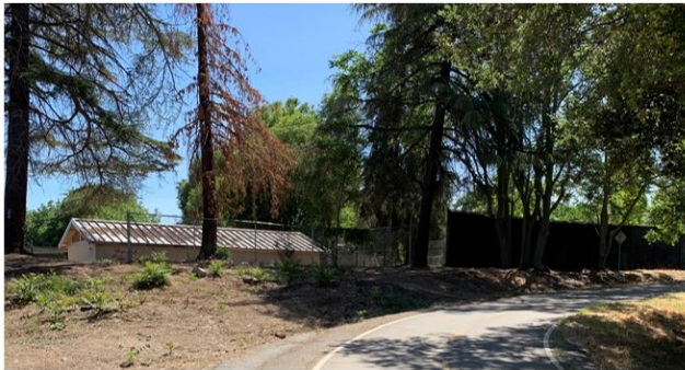
Fencing installations at Tully Minor Ballfield, including 150 feet along the foul ball line and a 70-foot perimeter enclosure, to deter encampments near Coyote Creek.
