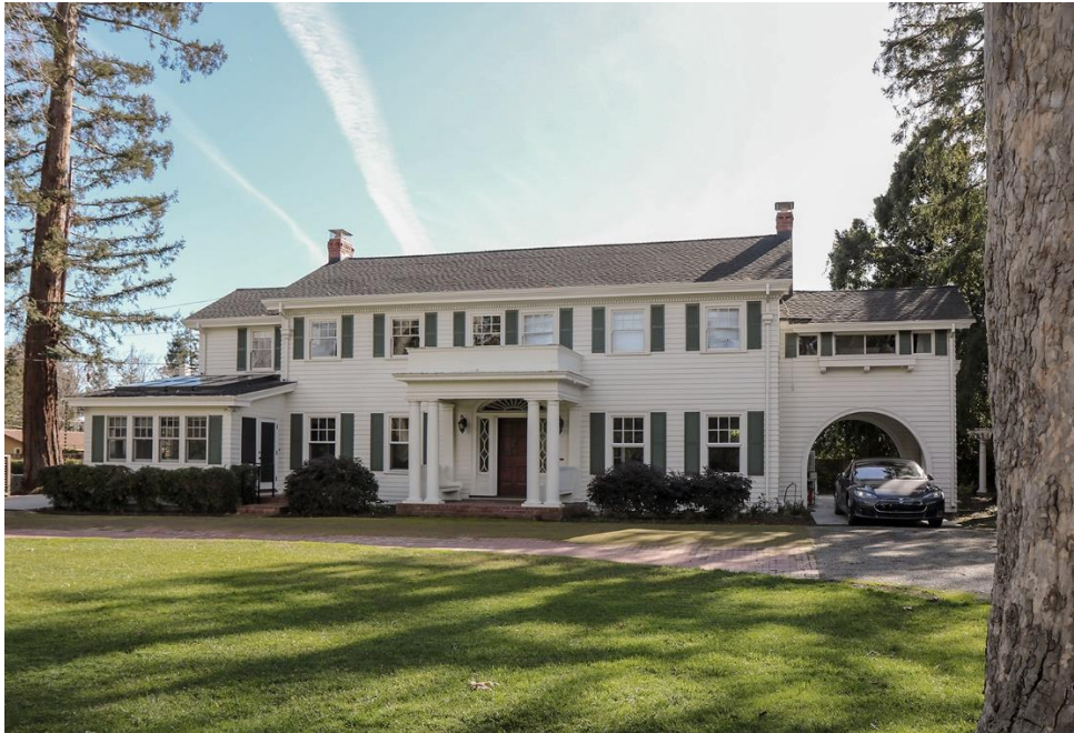
Front elevation viewed facing south-southeast. The distinctive porte-cochère with arched entrances is original to the house.
