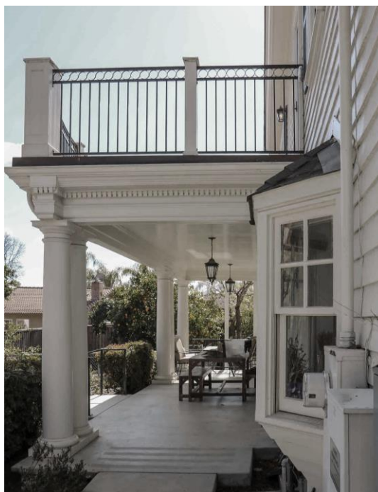
Side view of eastern wing.
