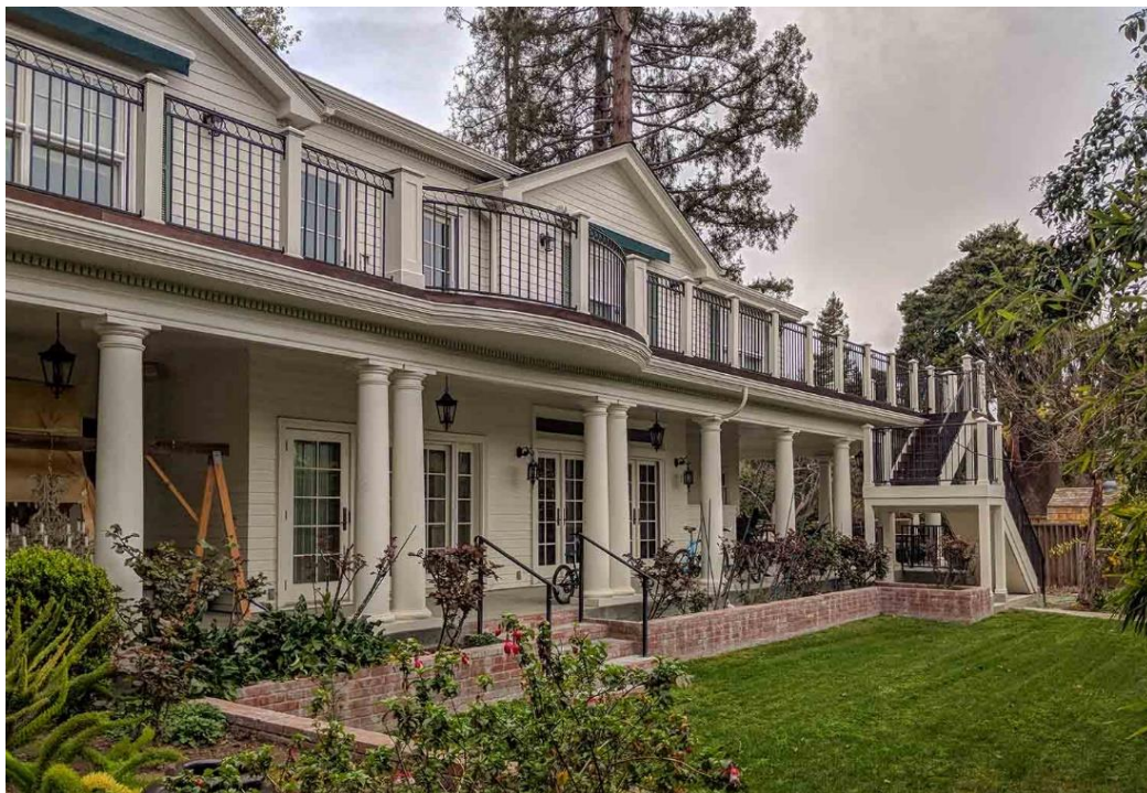
Back of house, view facing northeast, extension of house and added wraparound terrace and staircase.
