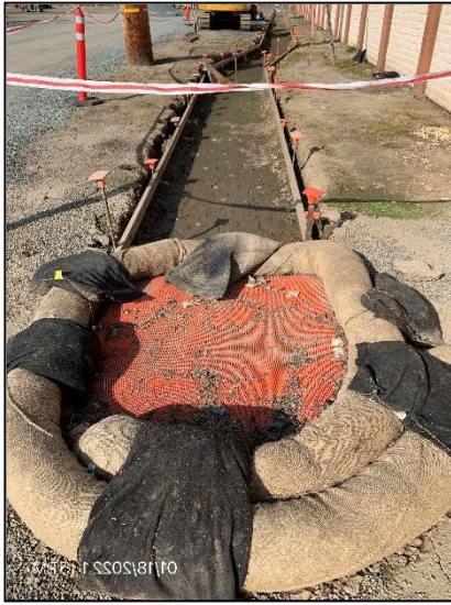
Effective BMPs installed at construction site.
